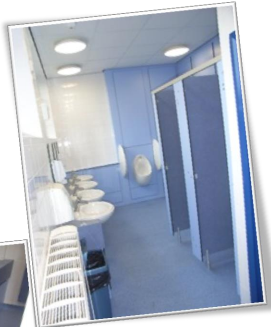
Toilet Refurbishment Works
