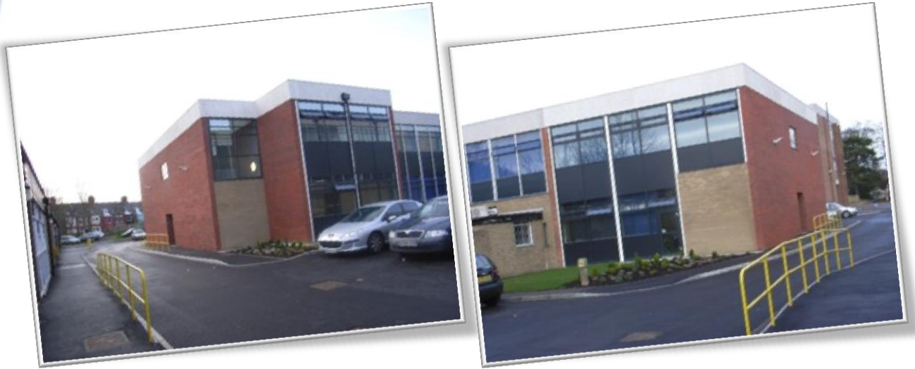
Block B Extension and Refurbishment - Completed and handed over from only a shell in 4 weeks
