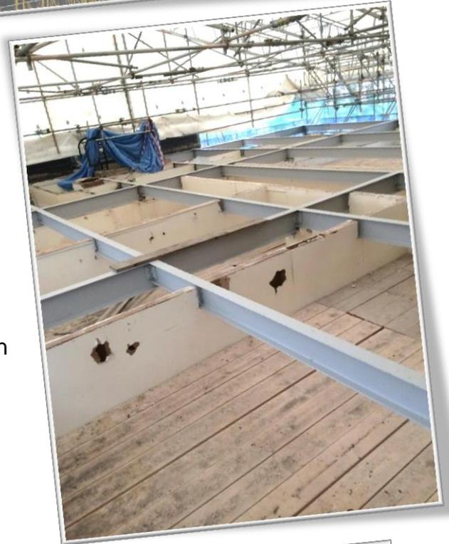
The building was enveloped with an over roof and sheeting to the facades to ensure that it remained watertight throughout the works. The parapets were then carefully dismantled and set aside for reuse, a scaffold crash deck installed inside the upper floor and the existing slab broken out in small sections and the steel frame repaired, before works could commence to reinstate/reconstruct the outer envelope.
