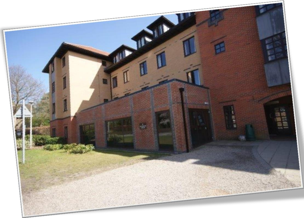
Library Extension to Holgate Building
