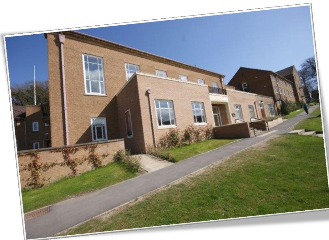
JCR Extension to Hollingside Building
