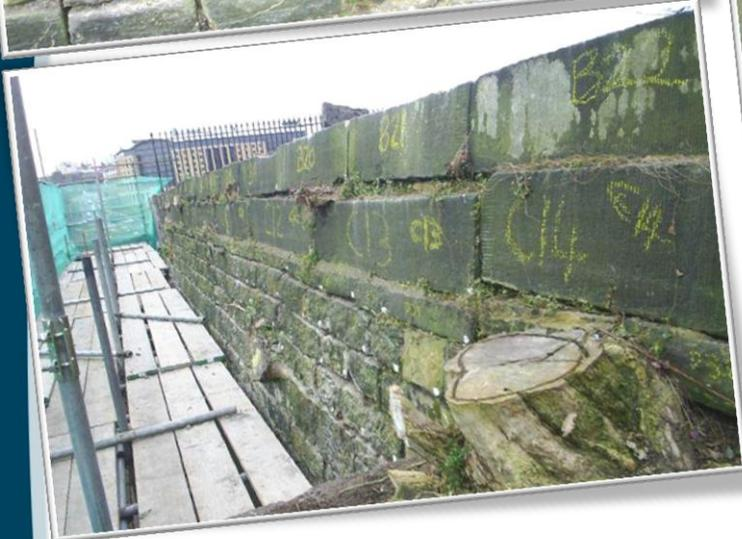
All of the stones were numbered and photographed to ensure that the wall could be rebuilt identically
