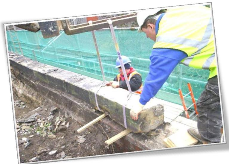
Many of the stones had to be carefully craned out of and back into position.
